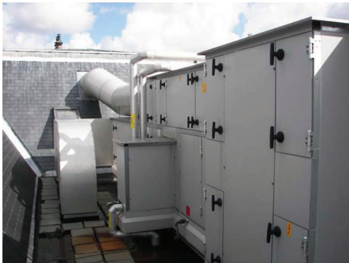
Figure 1. The air handling unit is placed on the roof.
